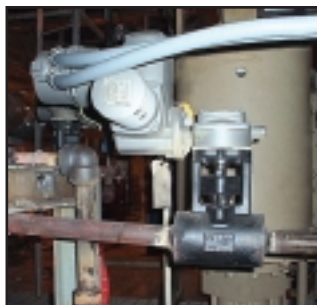
1 1/2" (40 mm) Power Ball Valves in steam trap isolation at a major British power plant. Switching to Velan Power Ball Valves offered a low torque, easy to operate solution.
