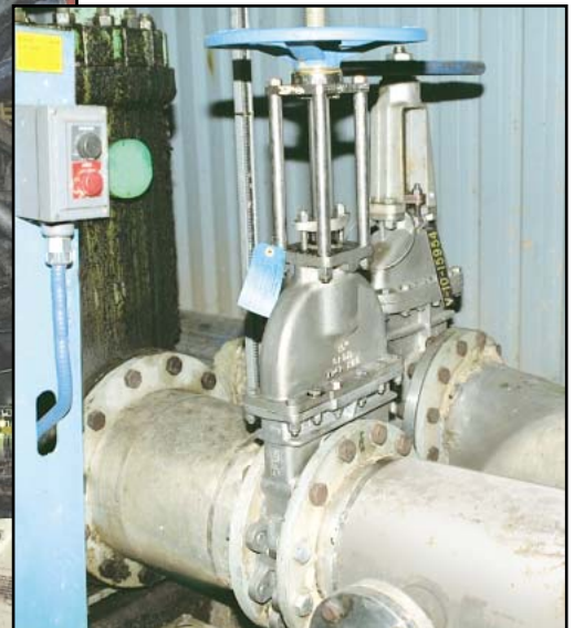
Filter isolation installation.
