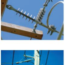
SILICONE COMPOSITE INSULATORS combine the technologies of a fiberglass reinforced rod, metal fittings and our extensive knowledge of elastomeric insulation to produce a high quality composite insulator. Since 1980, thousands of Silicone Insulators have been installed by utilities worldwide in a variety of environments. Continued outstanding performance is proof of their superior quality and design.
