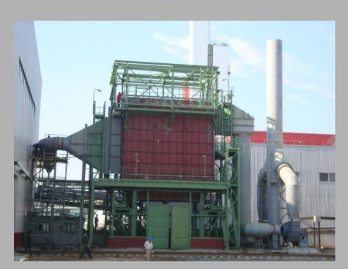
Italcementi Balikesir Cement Factory New Cement Mill Unit Bag Filter Fabrication and Erection Works (1x176.000m3/h, 1x60.000m3/h, 4x6.000m3/h)
