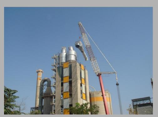
SItalcementi Ankara Factory Kiln No.2 Preheater Tower, Cyclones and Gas ducts
