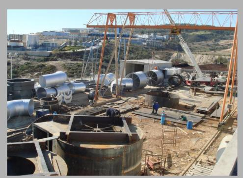
Italcementi Ankara Factory Kiln No.2 Preheater Tower, Cyclones and Gas ducts
