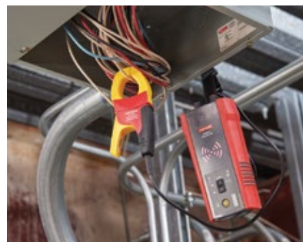
Sort bundled wires
