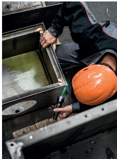
Dye penetrant testing
