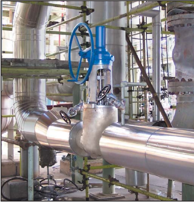
10" (250 mm) Pressure seal valve installed at Profertil's plant in Bahia Blanca, Argentina.
